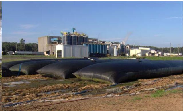
This food processing plant lagoon was pumped with a floating submersible pump pulled around to different spots with ropes. By moving the pump around most of the sludge was pumped over to the bags. Plastic Liner was used to divert the effluent that flowed from the bags back into the lagoon.
