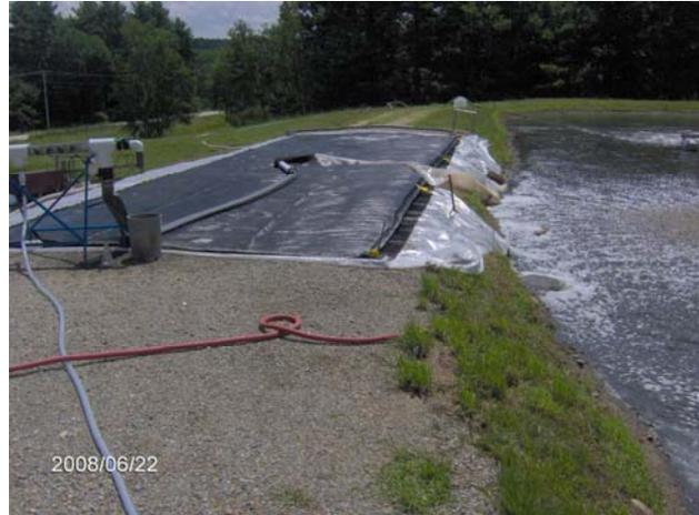
**This picture shows the results of having the proper chemical, injected into the line and properly mixed with the slurry. The solids have come together in clumps and the clear water surrounding the solids will simply exit thru the pores of the geotextile bag, leaving the solids behind. Keeping control of your process will greatly reduce the time needed for the sludge to dry and will reduce the overall cost of the project.**
