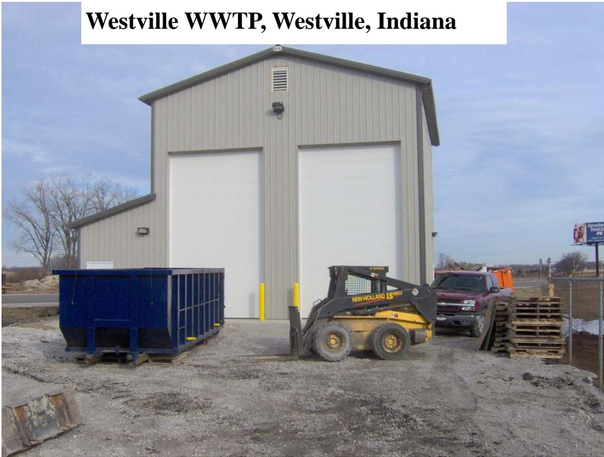
The town of Westville, Indiana built this building to hold two roll offs and also keep there polymer mixing and injection manifold inside for all weather dewatering. The building is 30' tall and the two overhead doors are 24' tall. The roll offs can be picked up and loaded inside the building
