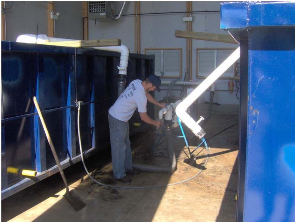
The operator has plenty of room between the roll offs to set up the mixing manifold. Future plans call for an overhead support to hold the fill tubes above the roll offs.
