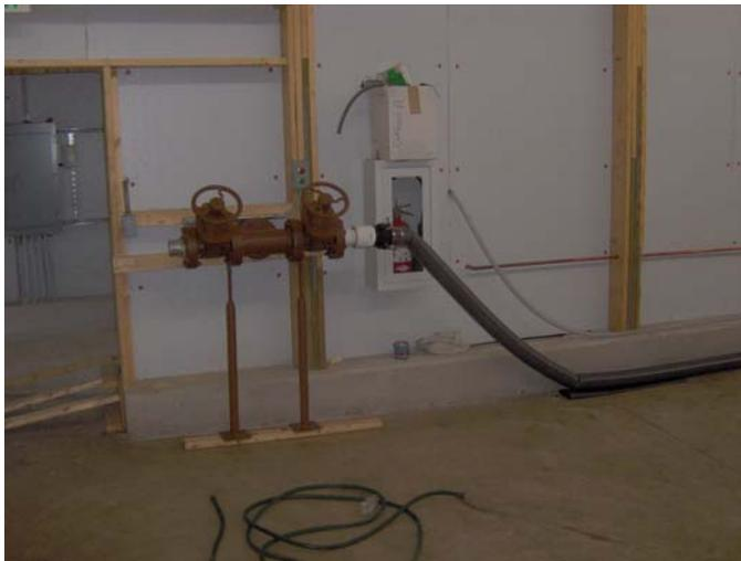
The sludge is pumped over into the roll off staging area and the two valves located on the wall are used to regulate the sludge flow as needed. The sludge is pumped over to a mixing manifold that is kept between the two roll offs.
