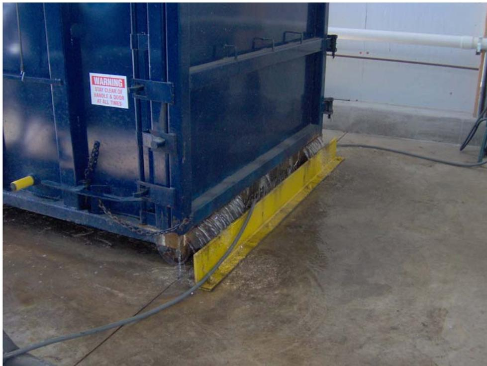
At the back of each roll off is an angle iron stop to facilitate the positioning of the roll offs. The effluent flows from the roll off into a drain where it is returned to the head works by a gravity feed drain pipe.
