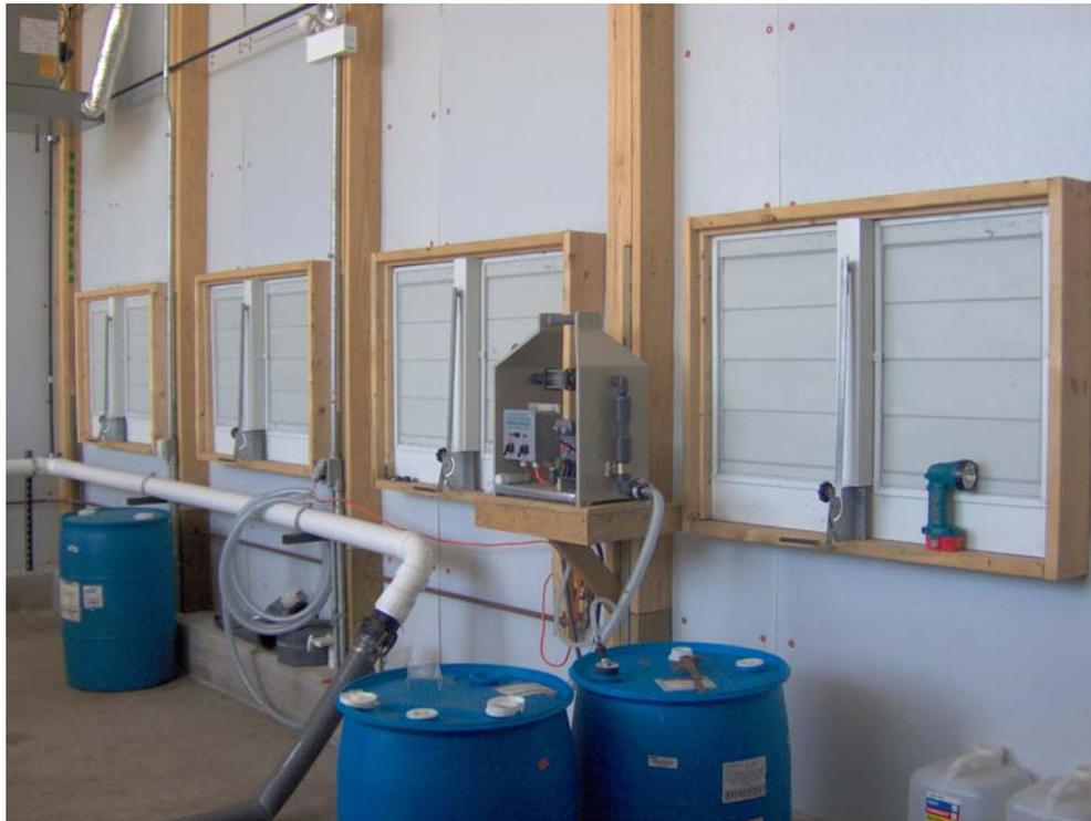
The sludge line is hard piped around the back wall. A cam lok fitting allows the operator to disconnect the sludge line easily. The polymer system is now located on the back wall for easy access.
