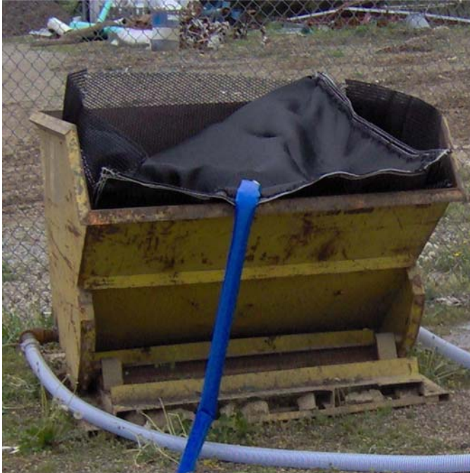
Installing the drainage netting
