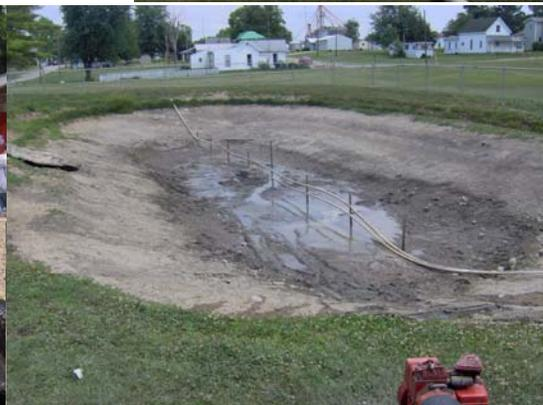
**Removing this lagoon sludge as a solid instead of liquid saved this small community thousands of dollars in cost.**
