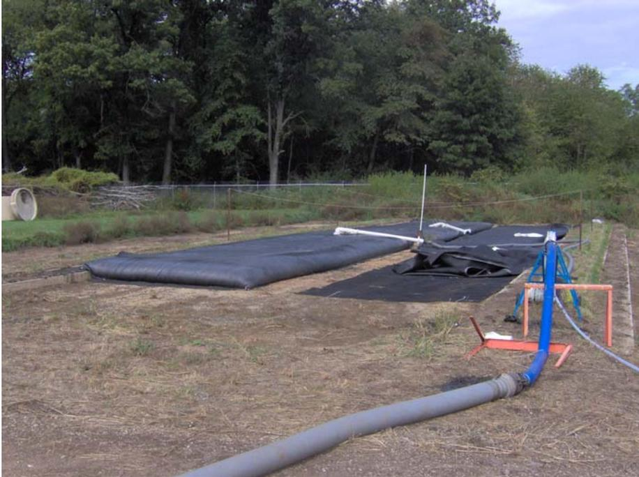
The pumping process begins. The 6" line running from the submersible pump over to the mixing manifold is used to reduce pressure drop as the distance from pump to manifold is fairly long.
