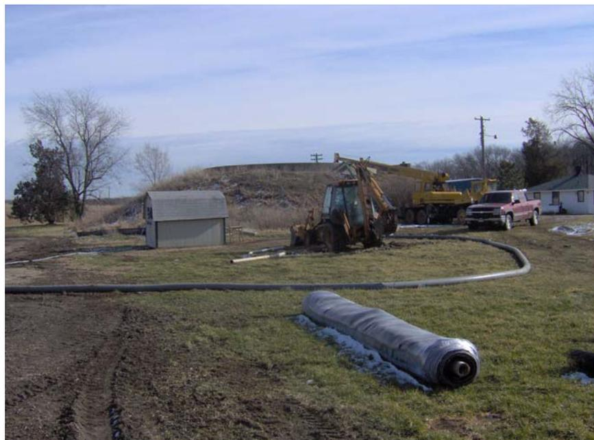
After cleaning out the beds, drainage mat was laid out over the clean sand. Two bags would be placed in each bed. The bags were Blue River Technologies 30' X 100' bags.
