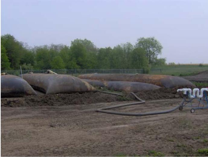
The digester was being filled with new septic waste as it was being pumped down so it took several months to pump it completely down and give it a much needed cleaning. To put the same amount of biosolids over the sand drying beds without the bags would have been impossible. The bags allowed the beds to hold many times more sludge than normal.
