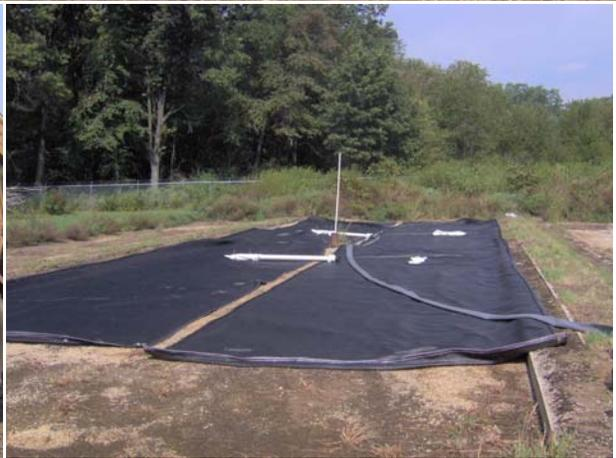
The bags were positioned on top of the drainage mat and rolled out to the full length of the bed.
