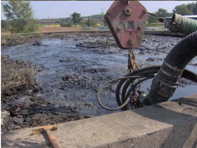
This old digester was completely full of bio-solids. Some of this waste had been in the digester for over 20 years and was heavily compacted in the bottom of the round concrete structure.
