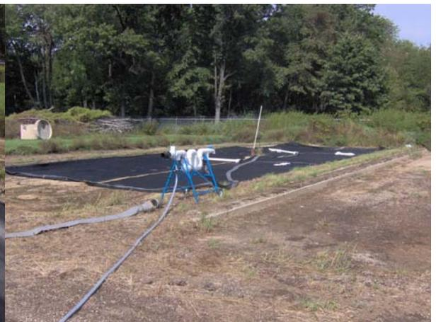
A pvc fill tube is placed into the fill port of each bag. The sludge mixing manifold is set up near the bags and a 4" hose used to connect the manifold to the bag. This hose is equipped with a camlok disconnect so that it can be switched from bag to bag as they are filled.
