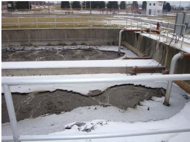
This picture shows the polymer mixing system and the flocculator. The sludge comes in from the left side, the polymer is injected and the sludge and polymer solution are mixed with the flocculator. A sample valve allows the operator to check the flocculated sludge from time to time.
