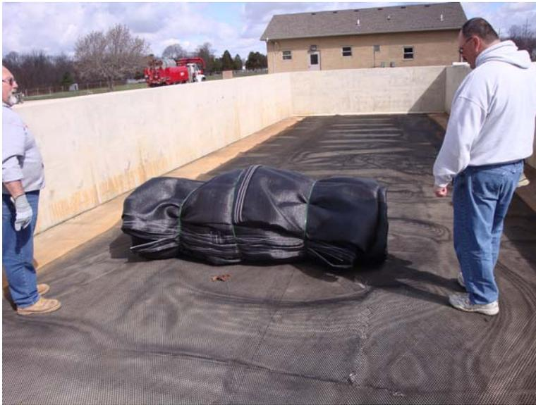
A new bag is rolled out over a drainage netting. This netting is reused over and over again and it helps the bag drain by keeping an air space between the concrete pad and the bottom of the bag.
