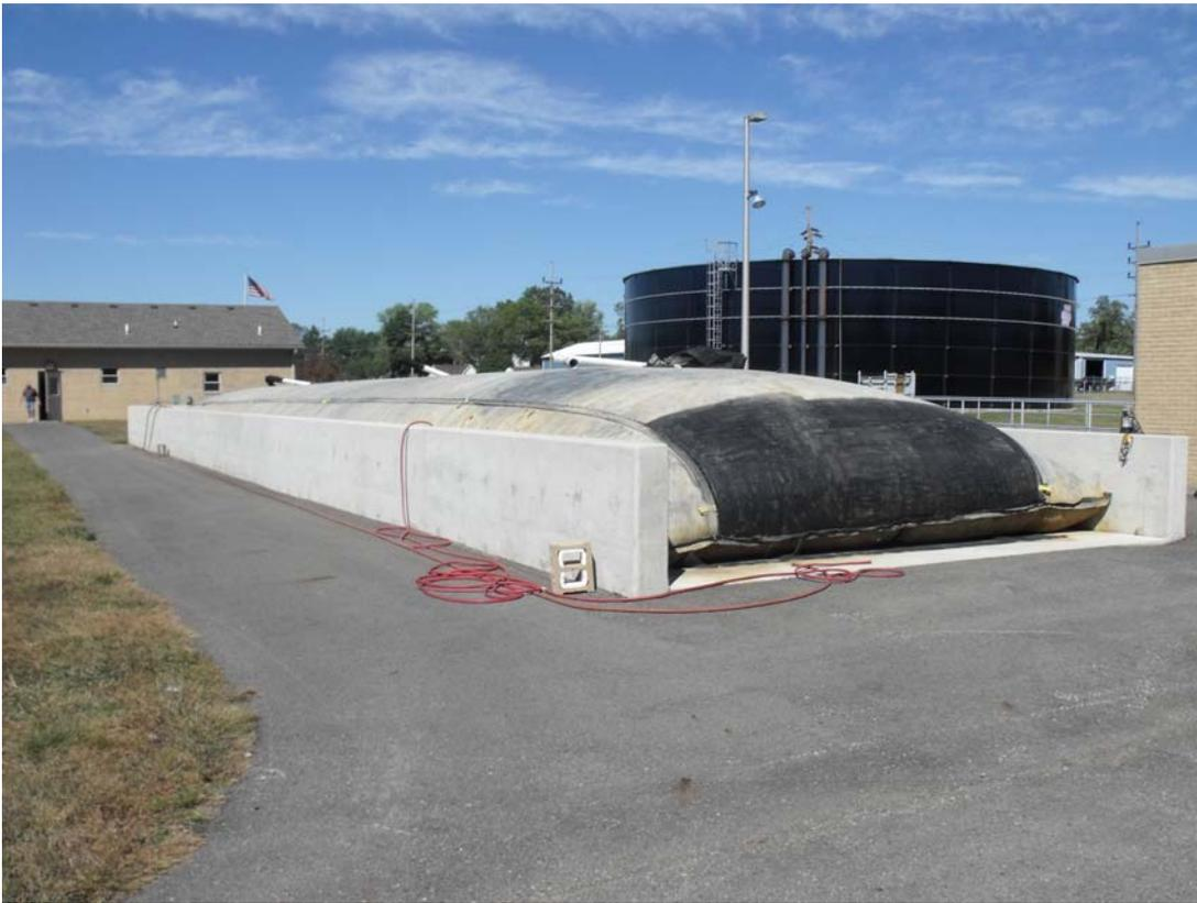
Gas City Indiana utilizes a 45' X 100' long geotextile dewatering bags to dewater approx 1,000,000 gallons of digested sludge per year. They fill and empty two bags per year, cutting open and land applying the solids in the spring and the fall when the farmer can get on the field. The bag is installed in a concrete bunker especially designed for the geotextile dewatering process.
